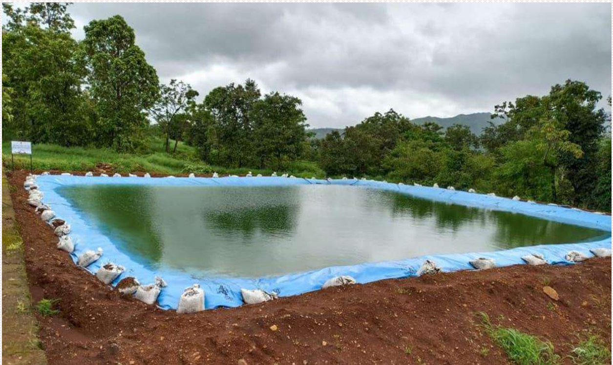
Figure 3: Ensuring availability of water through farm ponds with HDPE liner
